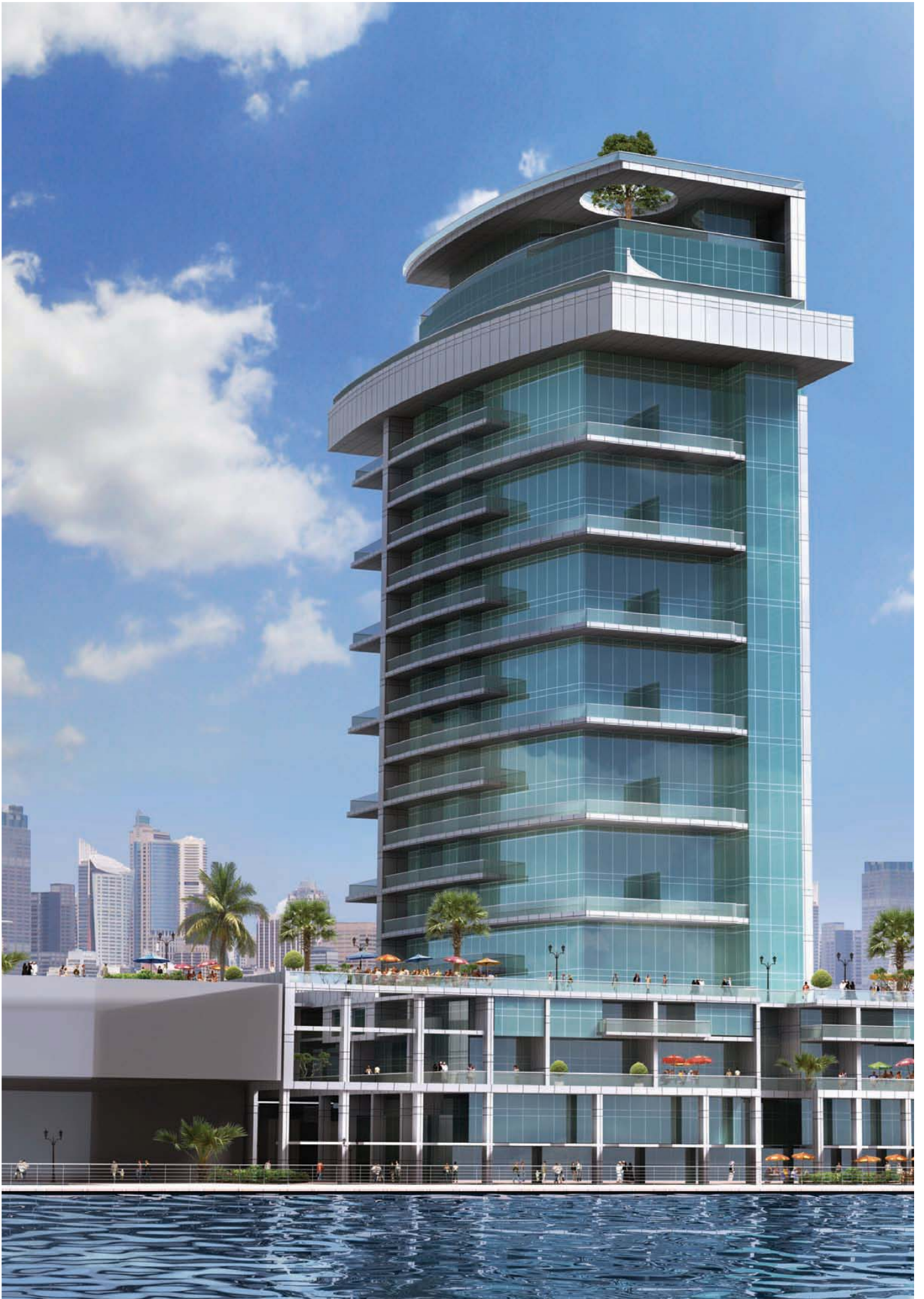
North elevation facing the Creek
